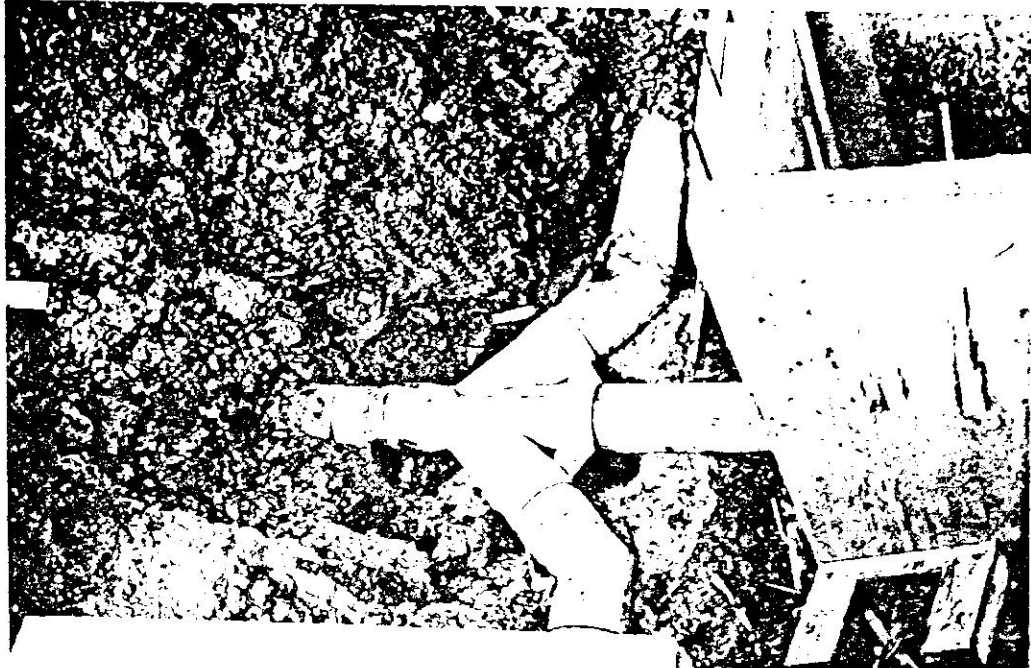
Figure 18. Pipe junction between the two digesters. Pipe from the mixing sump is to the left. The two branches go to the digesters, and the bypass to the pond is on the right.
